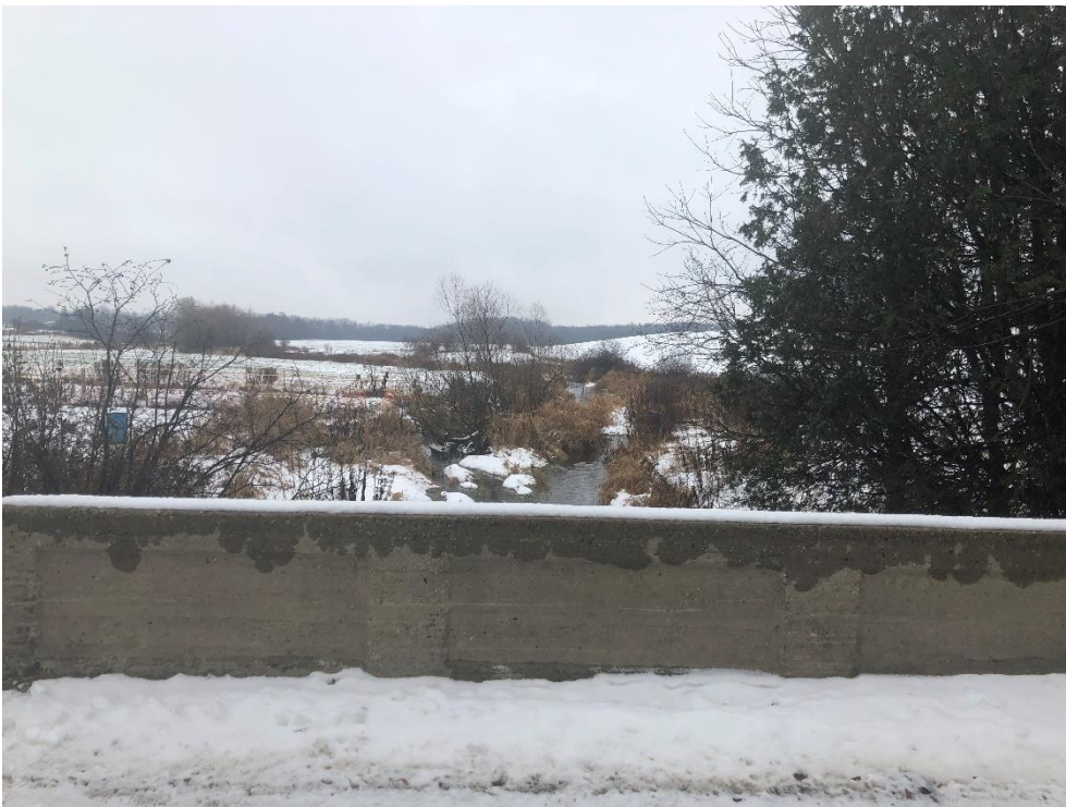
Plate 8: East parapet barrier looking east.
