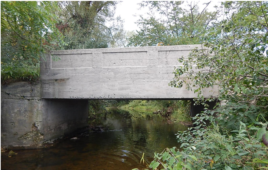
Figure 2: Photograph of the West Elevation of Structure 400172 ("Beitz' Bridge), ca. 2017
