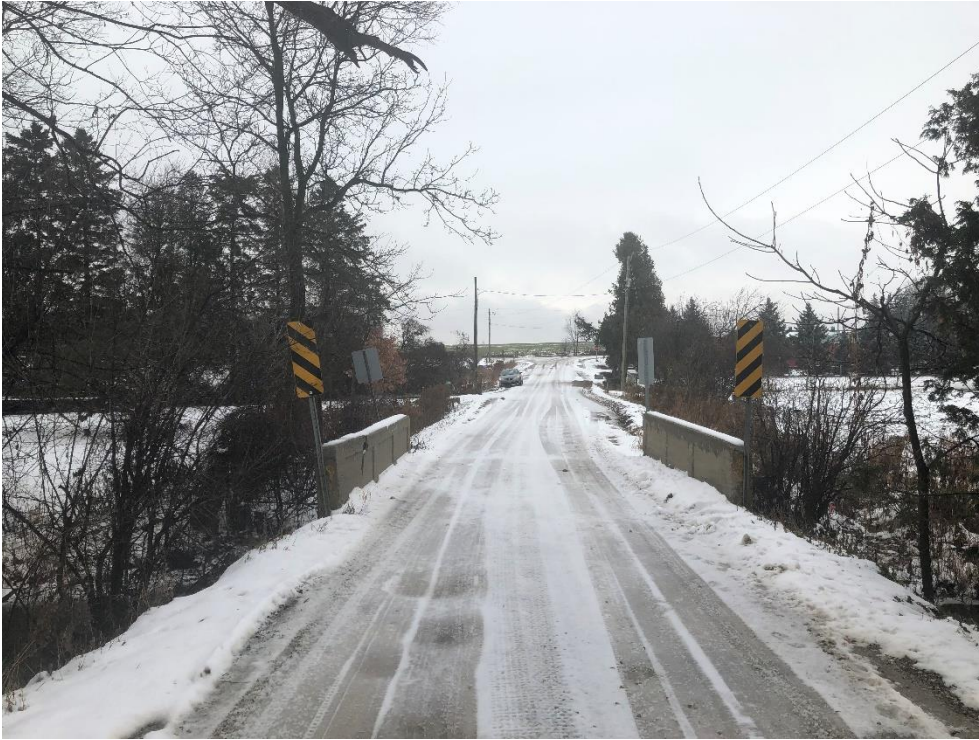
Plate 3: View of Structure 400172, looking south along Greenhouse Road.
