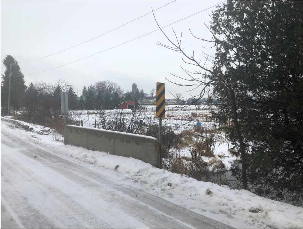
Plate 7: East parapet barrier.
