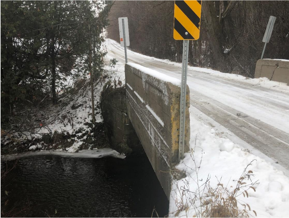
Plate 5: Oblique view of the bridge from the northeast quadrant.
