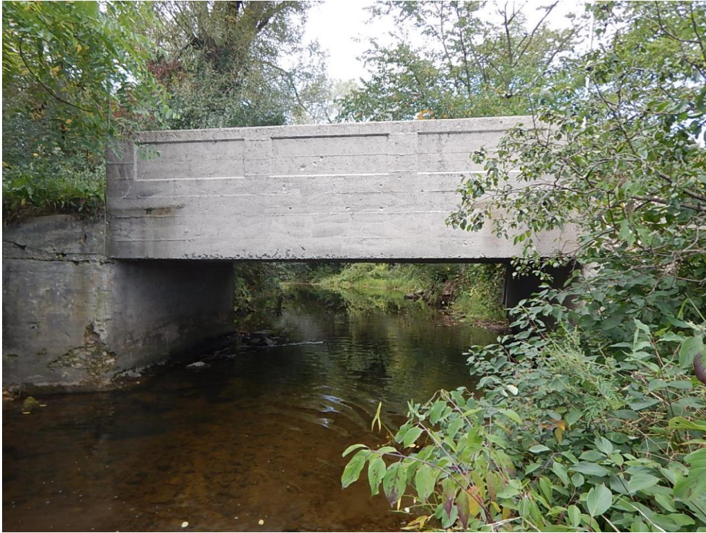
Figure 2: Photograph of the West Elevation of Structure 400172 ("Beitz' Bridge), ca. 2017 Source: Courtesy of GM BluePlan
