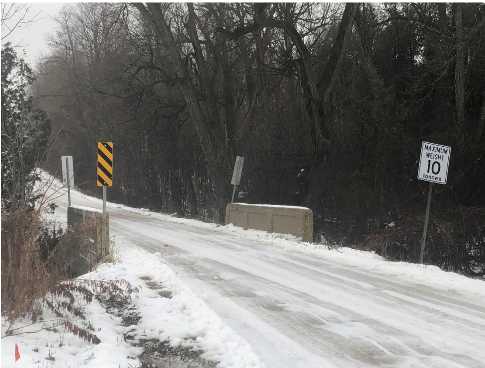
Plate 2: View of Structure 400172, looking southwest.
