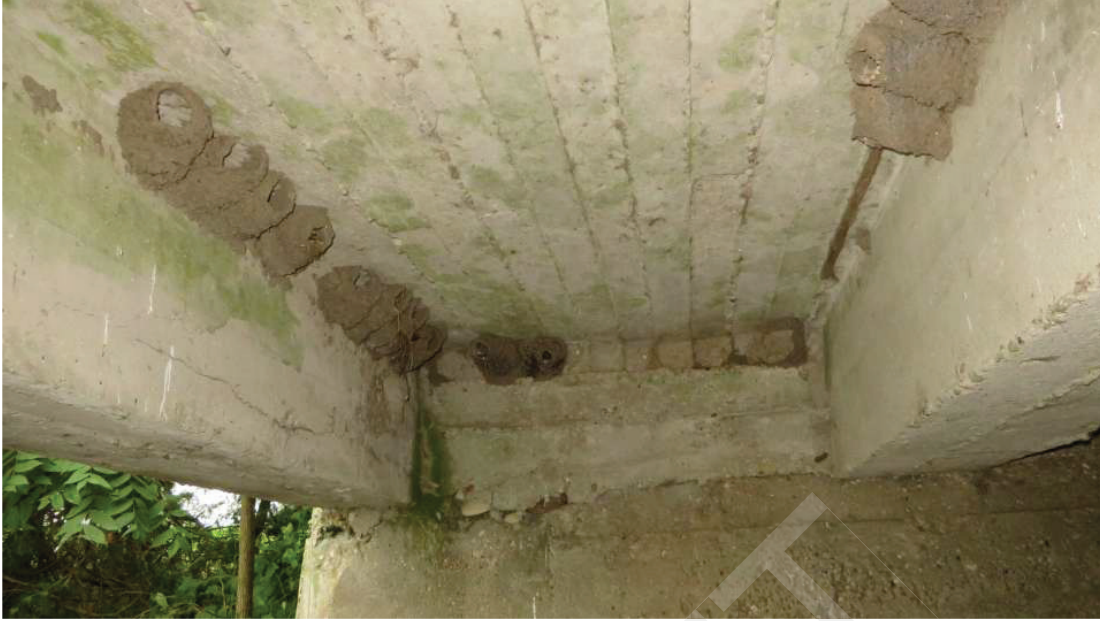
North girder end
