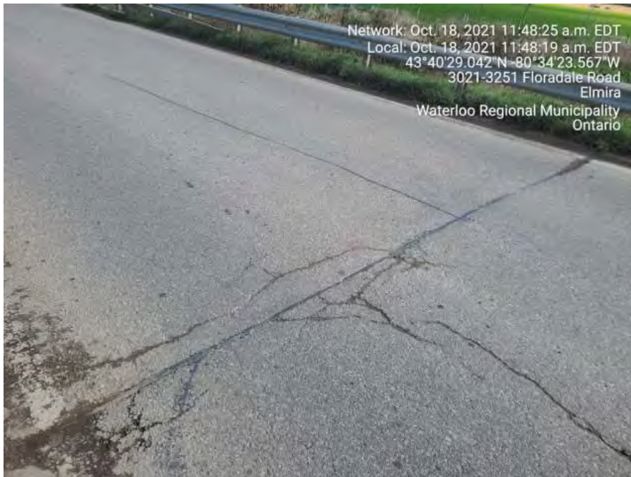
Wearing surface looking south
