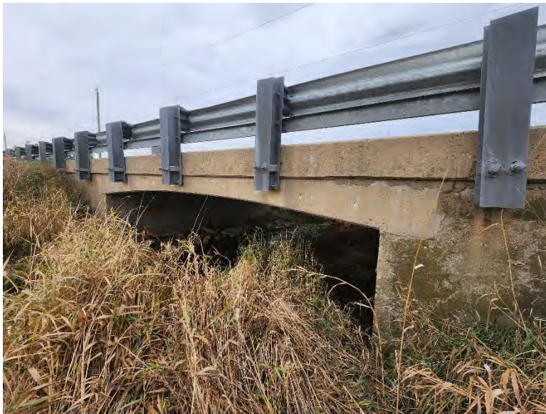
Figure 10: West elevation of the Floradale Road Bridge, looking northeast (A.S.I., 2022).
