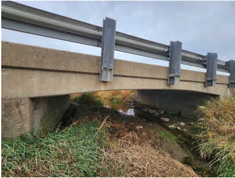
Figure 9: East elevation of the Floradale Road Bridge, looking west (A.S.I., 2022).
