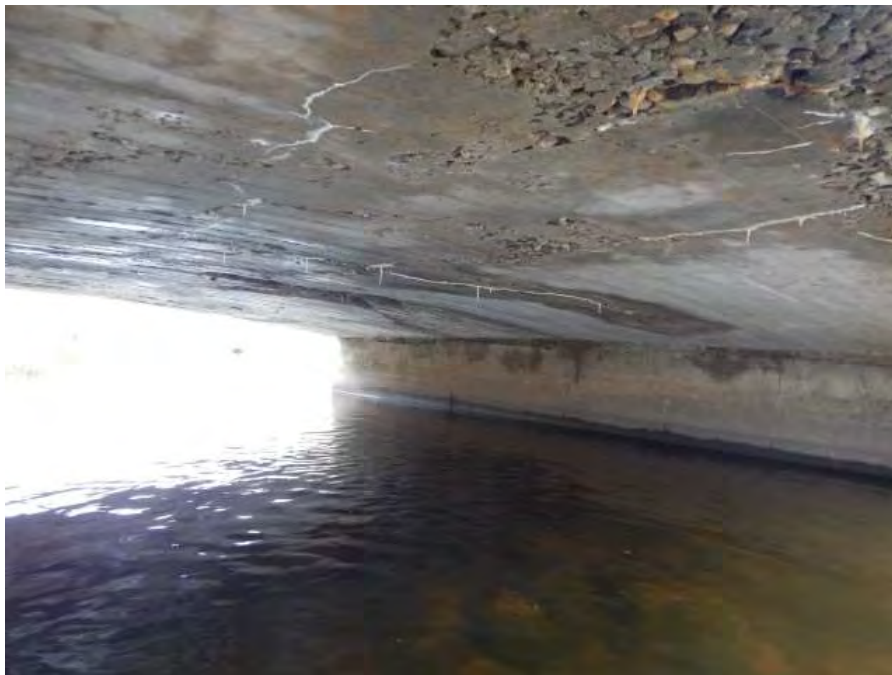
Soffit looking southwest
