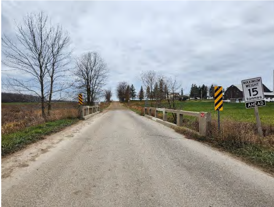
Figure 21: Nearby Spies Bridge (010105) on Sideline 18 with the original concrete barriers (A.S.I., 2022).
