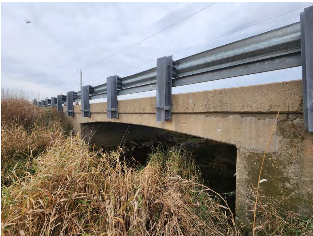
Figure 2: West elevation of the Floradale Road Bridge, looking east (A.S.I., 2022).
