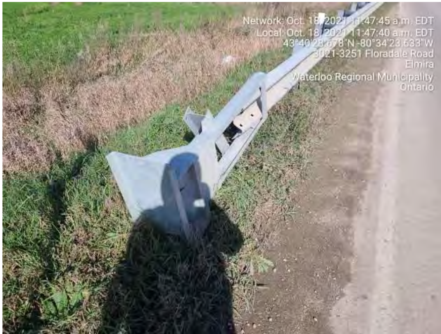
Southwest guide rail end treatment
