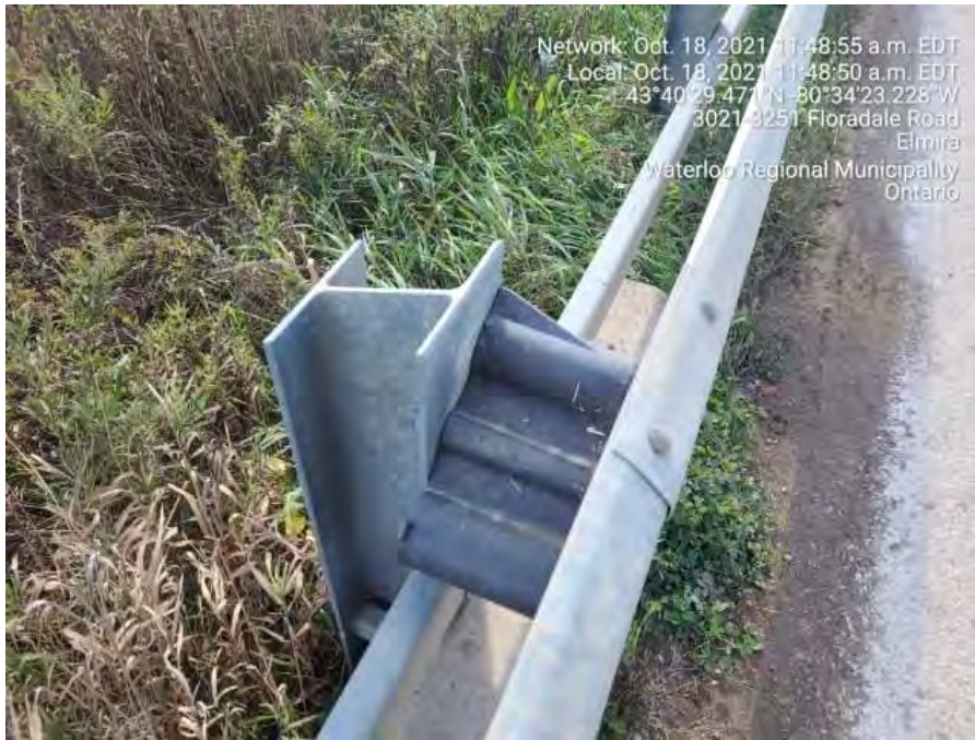
East guide rail showing a rotated offset block
