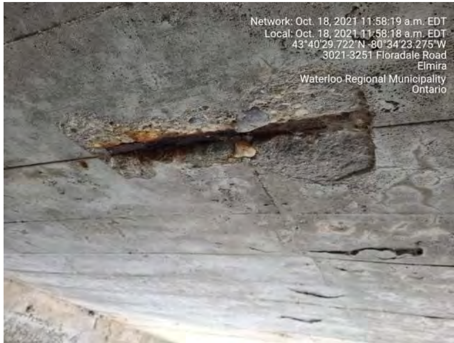
Soffit looking east showing severe spalling
