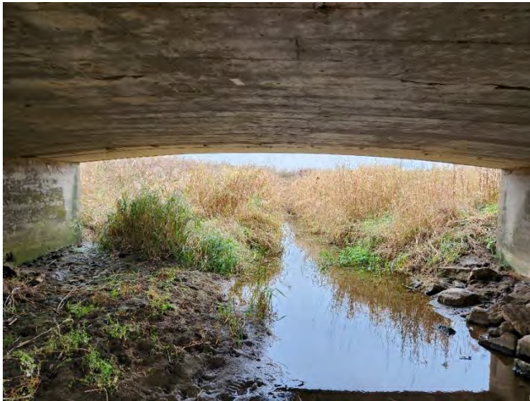
Figure 11: Detail view of bridge soffit and watercourse, looking west (A.S.I., 2022).
