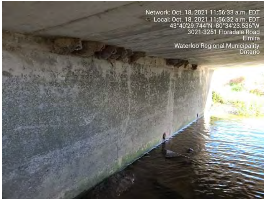
North abutment looking northeast
