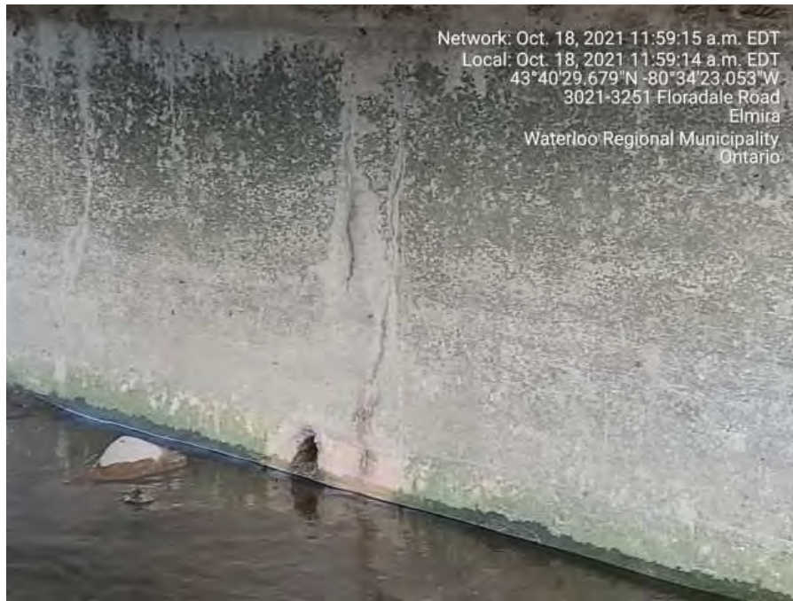
South abutment wall showing narrow vertical stained cracks
